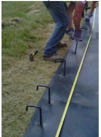
edge of the mat. Drill through the mat and into the ground the full 6 inches. This makes a good pilot hole for the anchor. Typically the anchor can then be forced through the mat into the ground 6 inches and then driven the rest of the way with a 6-8 pound hammer.
