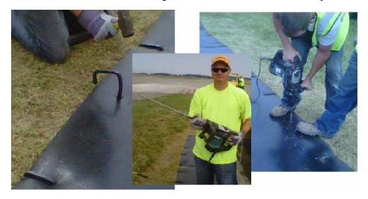
**Tools:** A line trimmer and blower for prep work where needed. A tape measure, razor knife, drill for starting anchors, A hammer drill for occasional trouble spot. And a hefty hand sledge is best for the stake anchors. Caulking gun and asphalt sealant (not provided). And Bring a Camera.\*
